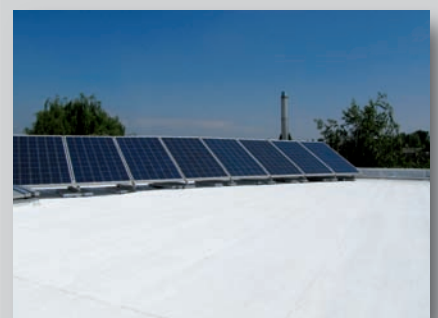
Finished Reflecta waterproofing system
