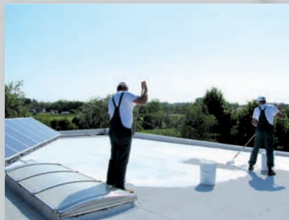
1st coating application
