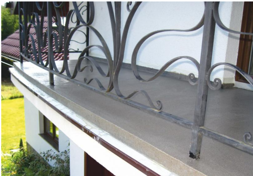
Balcony-epoxy floor, Banino
