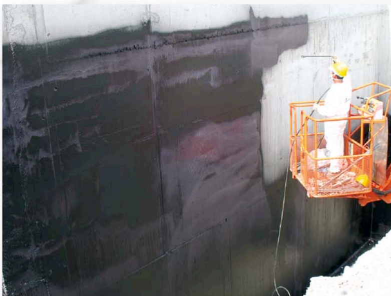
Waterproofing large surfaces
