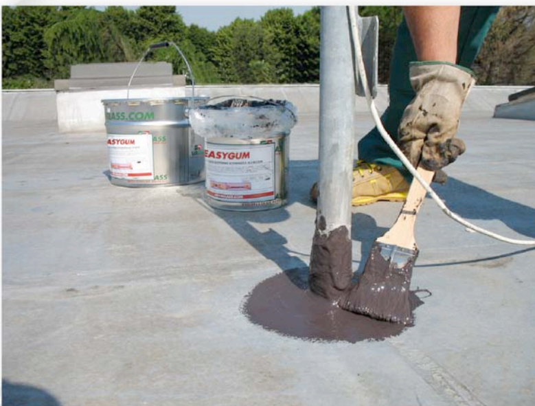
Restoration and ordinary maintenance
