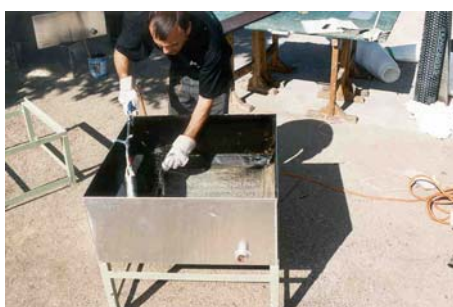
APPLICATION OF THE NOVAR-WS MEMBRANE ON THE WALLS OF THE CONTAINERS
